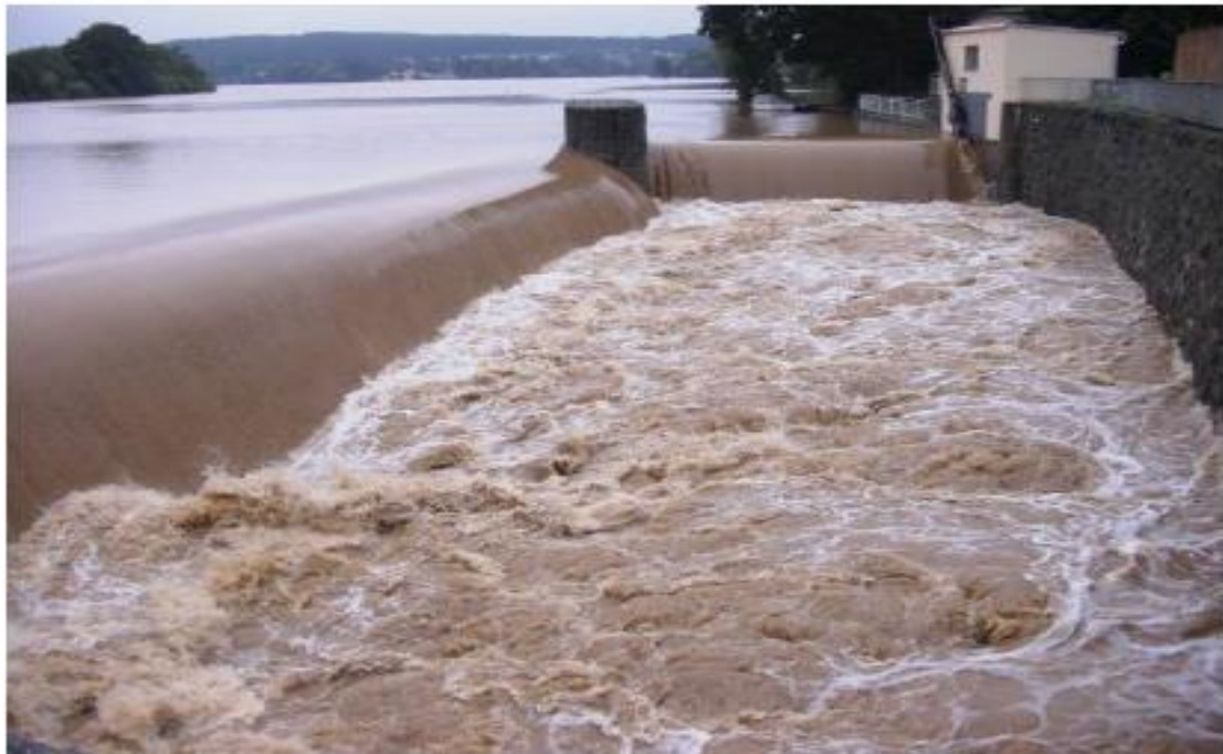
FIGURE 10. Side channel entry to a chute spillway
